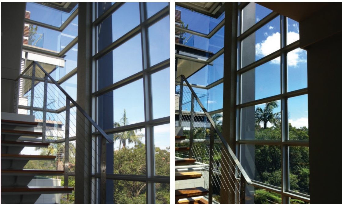
Before and After PR70
